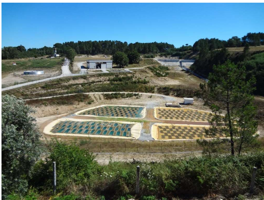
FIG. 2. Partial view of the old uranium mine site of Cunha Baixa, with the new water treatment station, water reservoir for irrigation, and passive water treatment ponds in first plane (View from the village, 2014).
